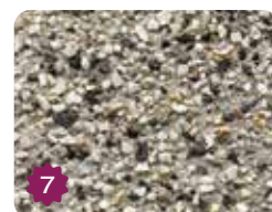
7 Driveway Boral Exposed Aggregate Daybreak
